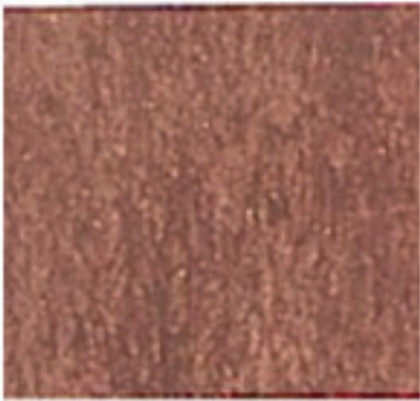
ASBESTOS JOINED SHEET
